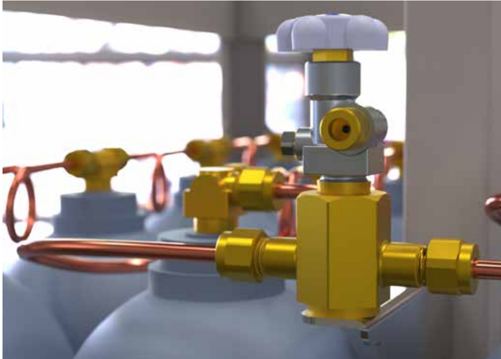
"RPV High Flow valve connected to the valve holder"
