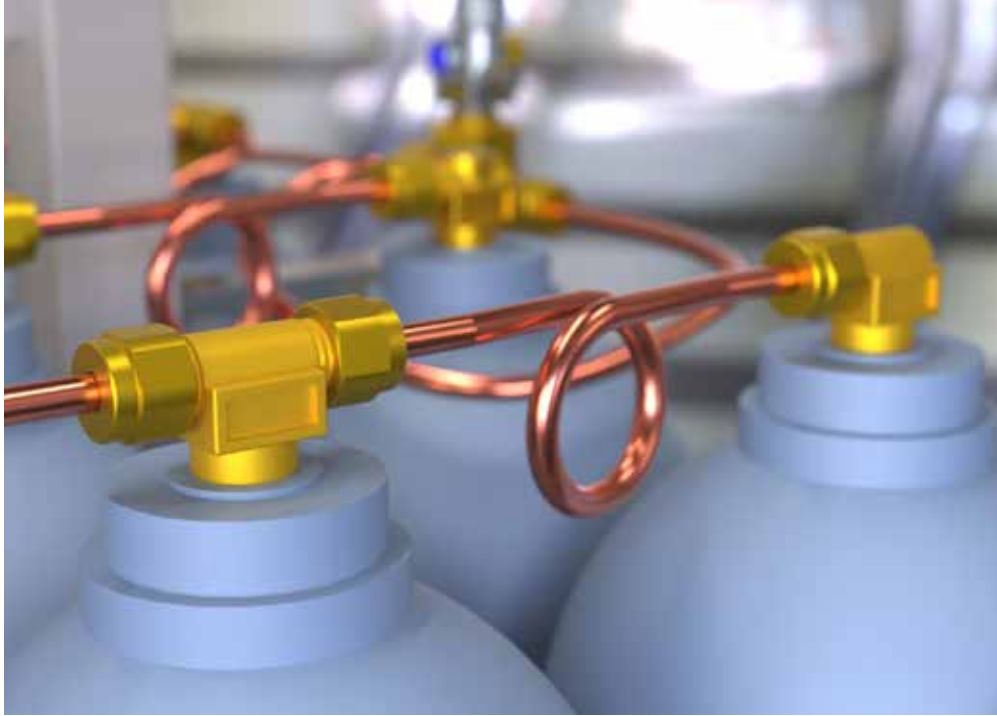
"A two way fitting linked to a one way fitting through a copper pipeline"
