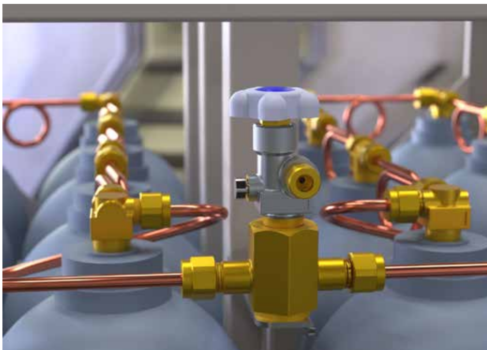
"The copper pipelines link the cylinders to the main valve through fittings and the valve holder"
